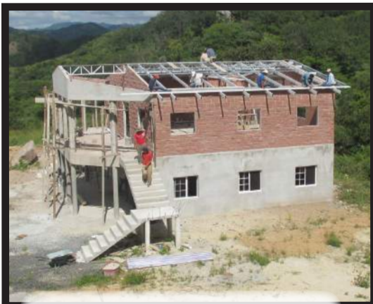
Construction of new Seminary Building
