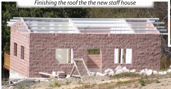
Finishing the roof the the new staff house
